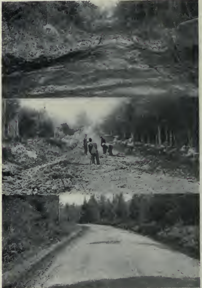
Good Roads in Compton, P.Q., Macadam built in 1915, Road before, during and after construction.
